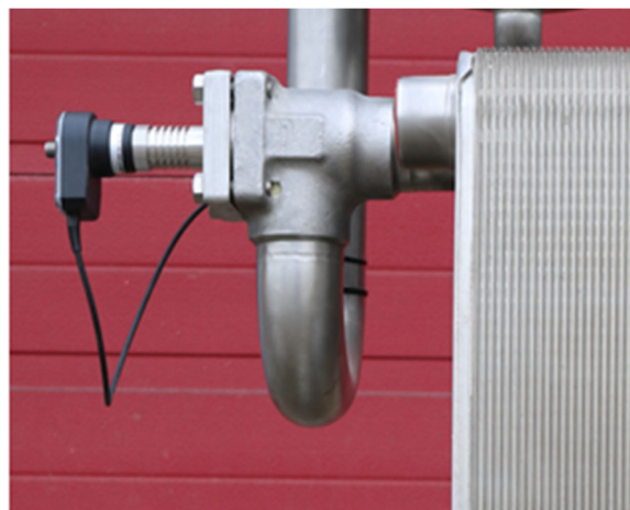
HBX sensor in strainer housing used as leakage detector installed after plate heat exchanger
